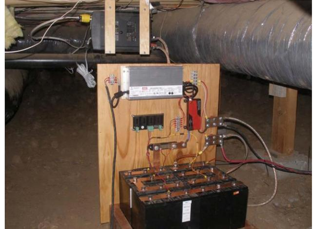
It has 540 A/H of LiFePO4 battery storage, a 35 amp charger, 600 watt sinewave inverter, and 3 x 100 watt solar panels. It lives in the crawl space under the hamshack and was completed 15 minutes AFTER (with headlamp) the last PG&E PPS event began. It normally powers the shack, but will run the kitchen refrigerator for 4 days if I stay off the air
