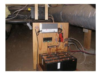
It has 540 A/H of LiFePO4 battery storage, a 35 amp charger, 600 watt sinewave inverter, and 3 x 100 watt solar panels. It lives in the crawl space under the hamshack and was completed 15 minutes AFTER (with headlamp) the last PG&E PSPS event began. It normally powers the shack, but will run the kitchen refrigerator for 4 days if I stay off the air
