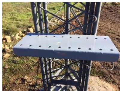
After getting the shelf level and installed it was a simple matter to install the winch on the shelf. Before bolting it down to the shelf though I had to take the hoist motor/reel off its frame to install the tower cable.
