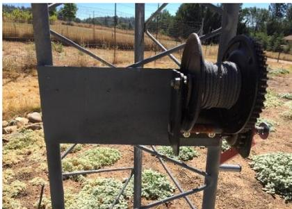
After cranking down the tower, removing the cable from the winch and removing the winch from the tower plate I could install the shelf to determine where I needed to drill two holes on the left of the tower plate. There are a total of five bolts holding the shelf to the tower plate.
