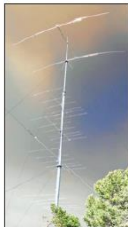
This is a 125-foot monopole with four stacked six-element, 10 meter Yagis and a two-element 40 meter beam.
